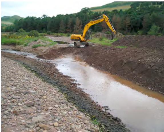
Figure 26: Bowmont Water channel dredged 05 August 2009 approx 1m below natural bed level.
